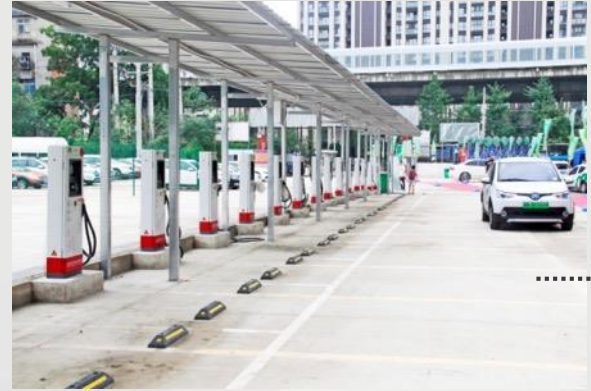
Super Charging station in Wuhan
