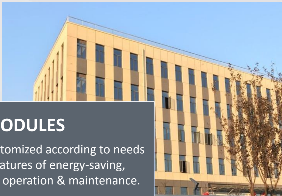
43 sets micro-modules for China Telecom (Jishan) Data Center Phase I.
